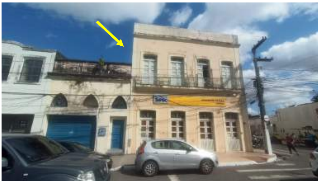
12 Prédio Principal – Fachada principal (Rua Augusta)
