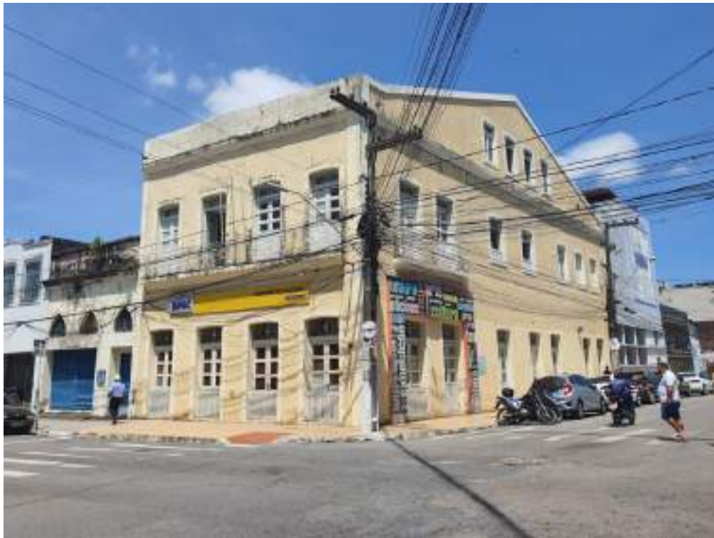
03 Fachada principal (Rua Augsuta)
