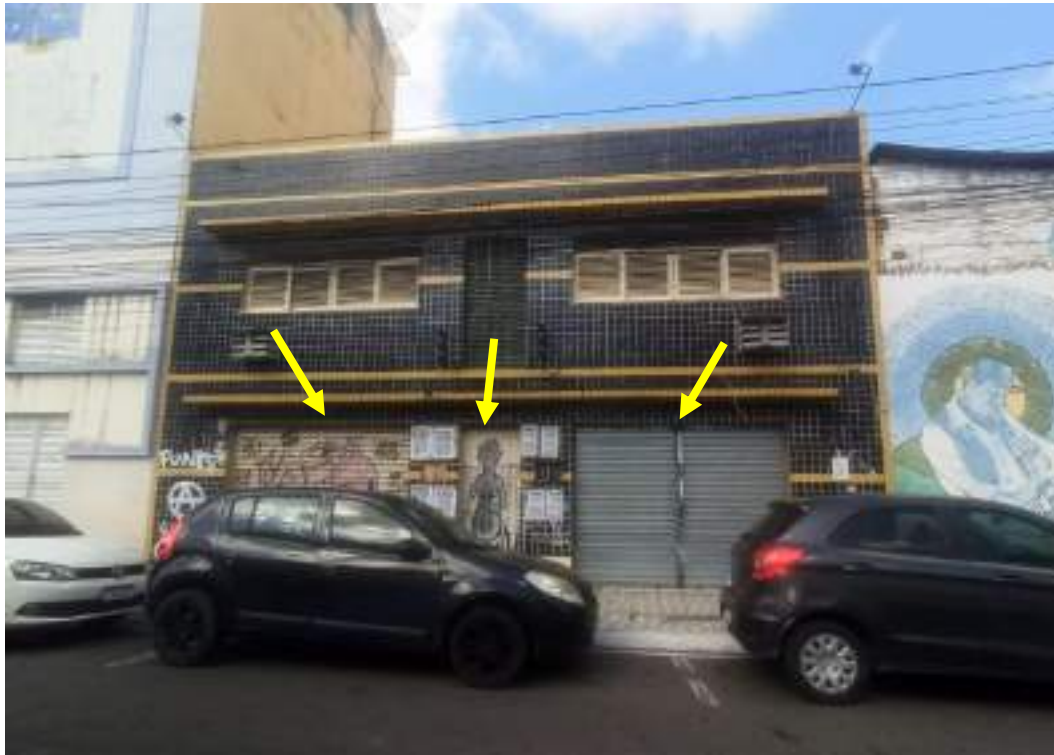
72 Fachada principal (acessos)
